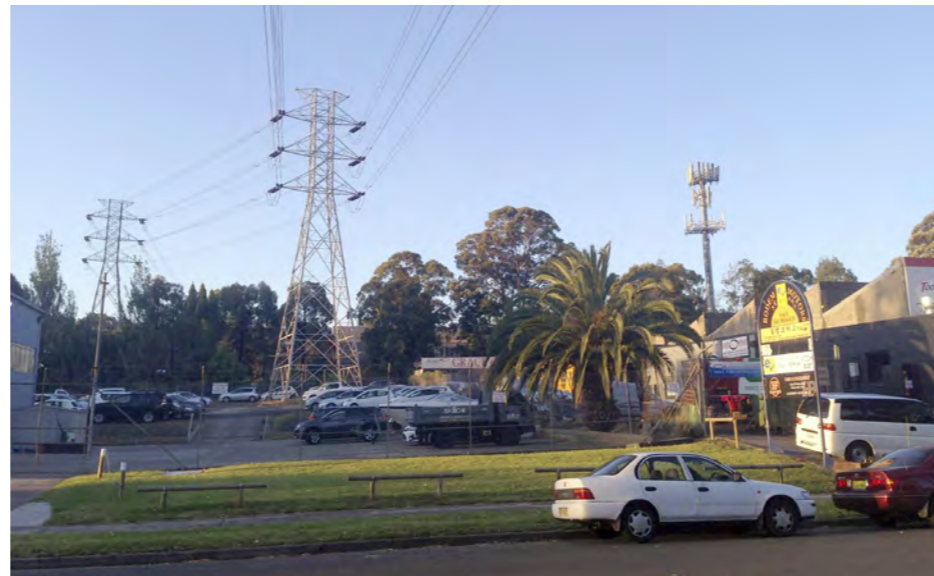
View 5 - Looking north from Hope Street at existing industrial around The Site and the high voltage power lines running along the western end of the Site.
